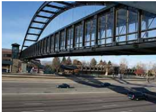
An example of light-rail access over a freeway, from Denver's Southeast Corridor.
